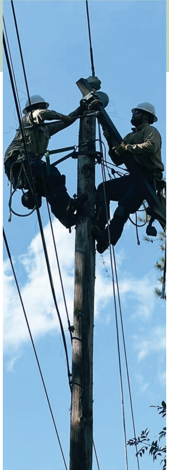
In the aftermath of Hurricane Helene, Fairfield Electric's Dustin Duggins and Xan Johnson teamed up to change a crossarm on a three-phase pole. Our linemen worked diligently to restore power.
